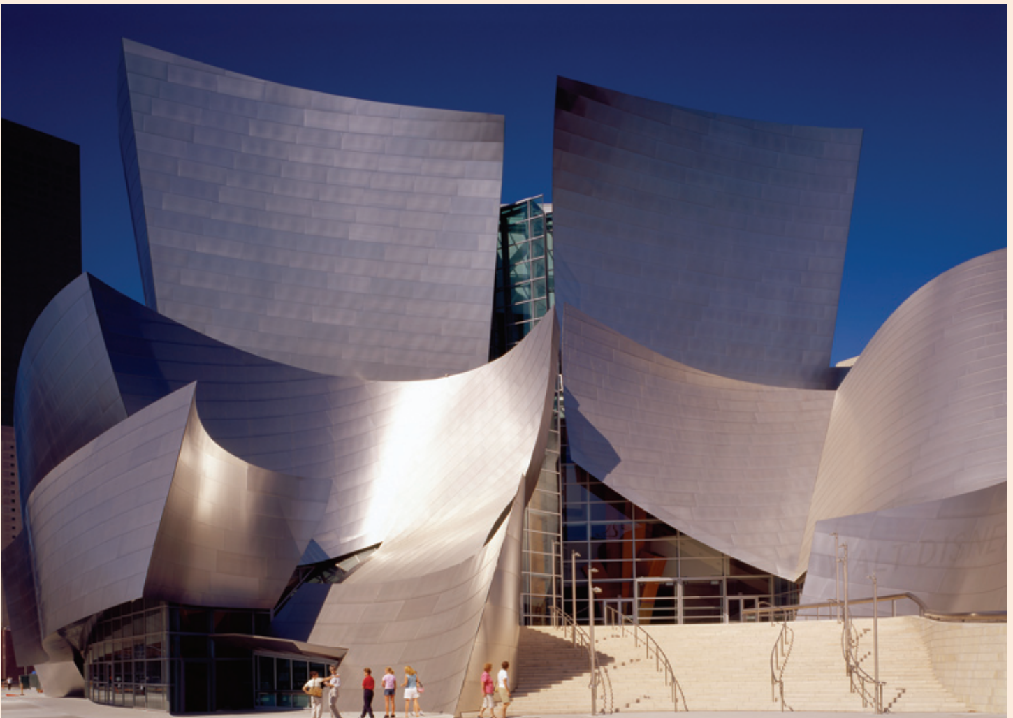
Photo: M. A. Mortenson Company, Lara Swimmer Photography
